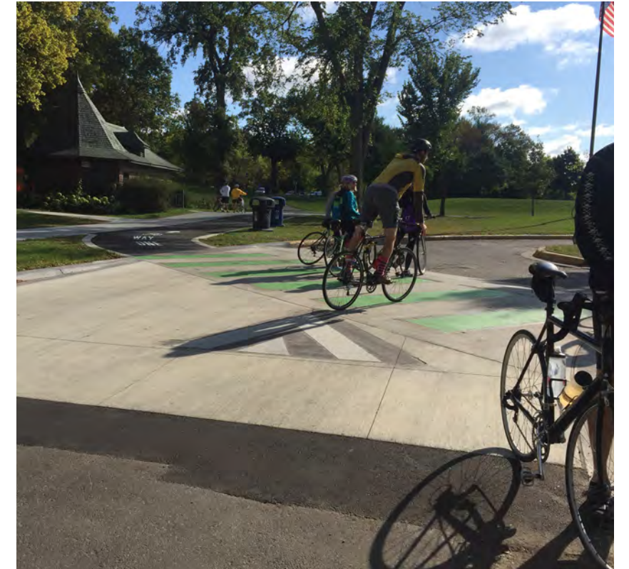
Raised Trail Crosswalk (Minneapolis, MN)
