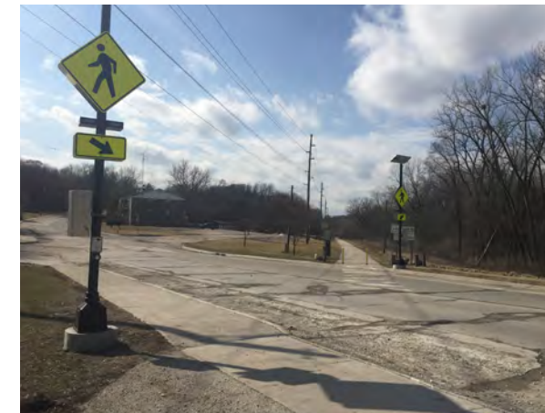
Flashing Beacons at the intersection of the Fort Dodge Nature Trail and Williams Drive. (Fort Dodge, Iowa)
