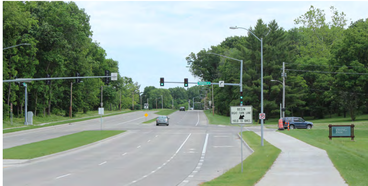
Sidepath trails may be supplemented by an on-street bicycle facility. This allows pedestrians and slower cyclists (e.g. children) to use the sidepath, while faster cyclists may choose to bike on the street. (Indianola Ave., Des Moines, IA)
