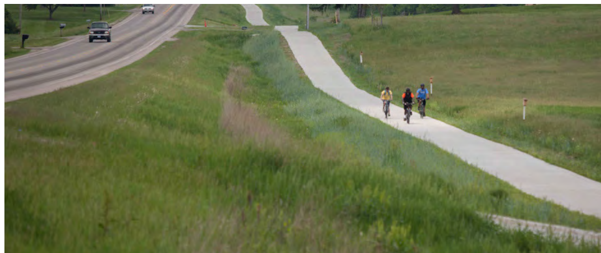
Sidepath trails may be appropriate along rural roadways with a few low-volume driveways or intersections. (Gay Lea Wilson Trail)
