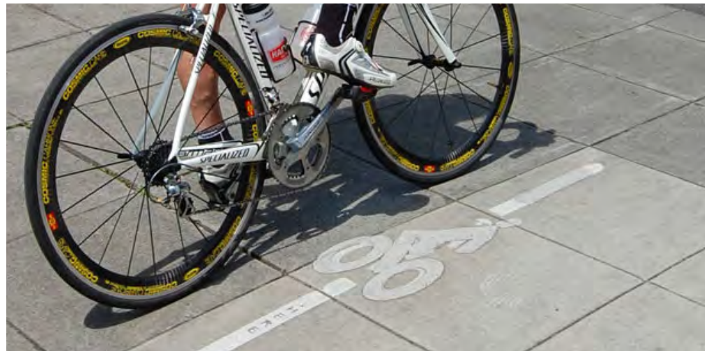
Loop cycle detector (Portland, OR) Source: (Urban Bikeway Design Guide, NACTO)
