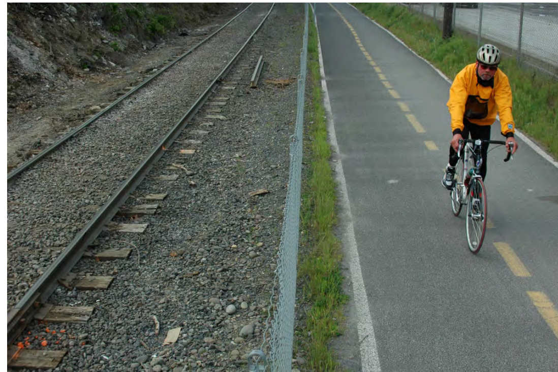
“Rail with Trail” facility using a chain link fence as a barrier (P)
