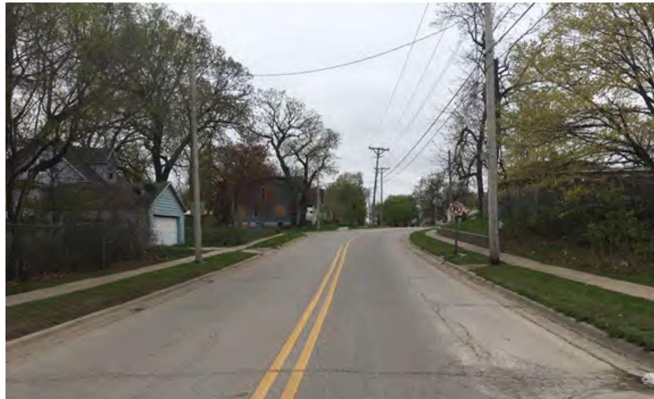
Roadway provides sidewalks, but no bicycle facility.
