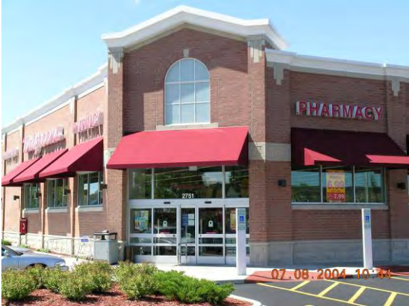
Public entrances should be articulated from the building mass using such means as a raised parapet and distinct tile work.
