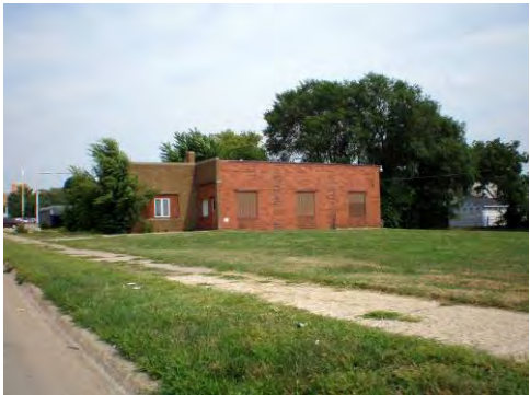
Undeveloped parcels create opportunities for land assemblage and redevelopment.
