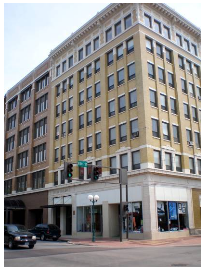
Downtown’s historic fabric is a major asset that can draw local and regional interest.
