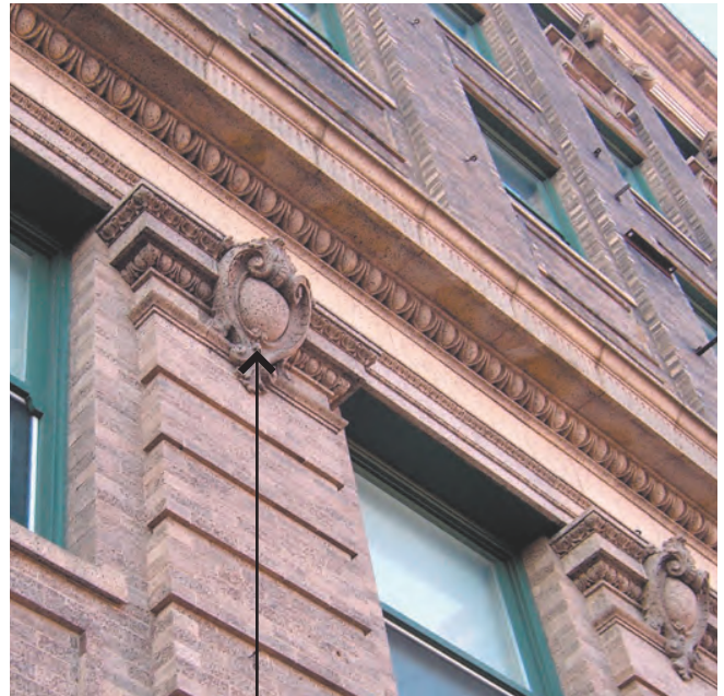
C Decorative masonry elements (columns, caps and cornices)
